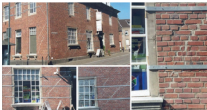
Fig. 3. Damage caused by surface uplift following mine-water flooding (12).
